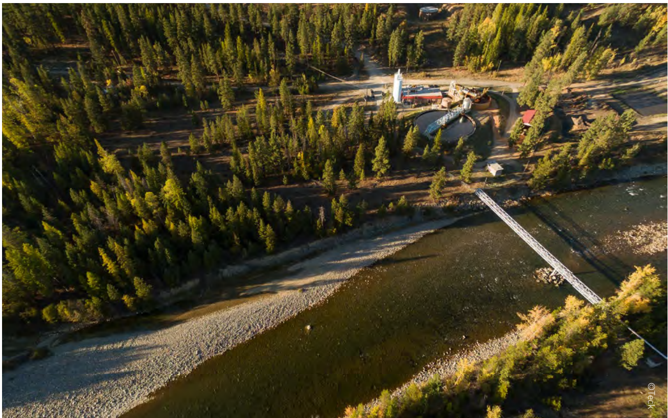
Water treatment plant at closed Sullivan mine, Canada
