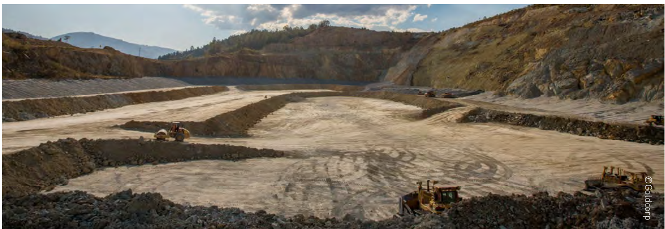
Open pit backfilling at Marlin Mine, Guatemala
