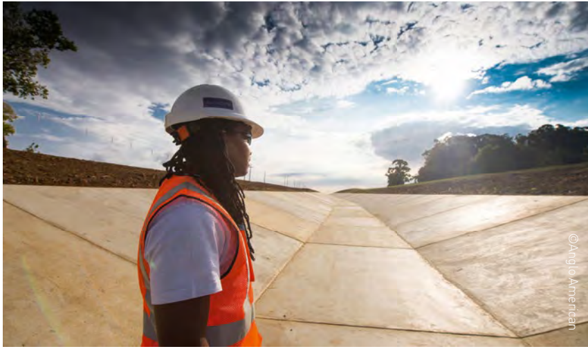
River diversion at Isibonelo Colliery, South Africa
